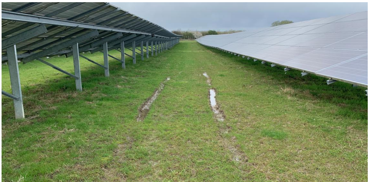
Plate 11-41 Example of Minor Ruts Caused by Vehicles
