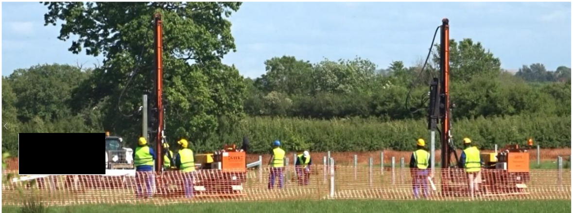
Plate 11-27 Mounting Structure Piles being Installed
