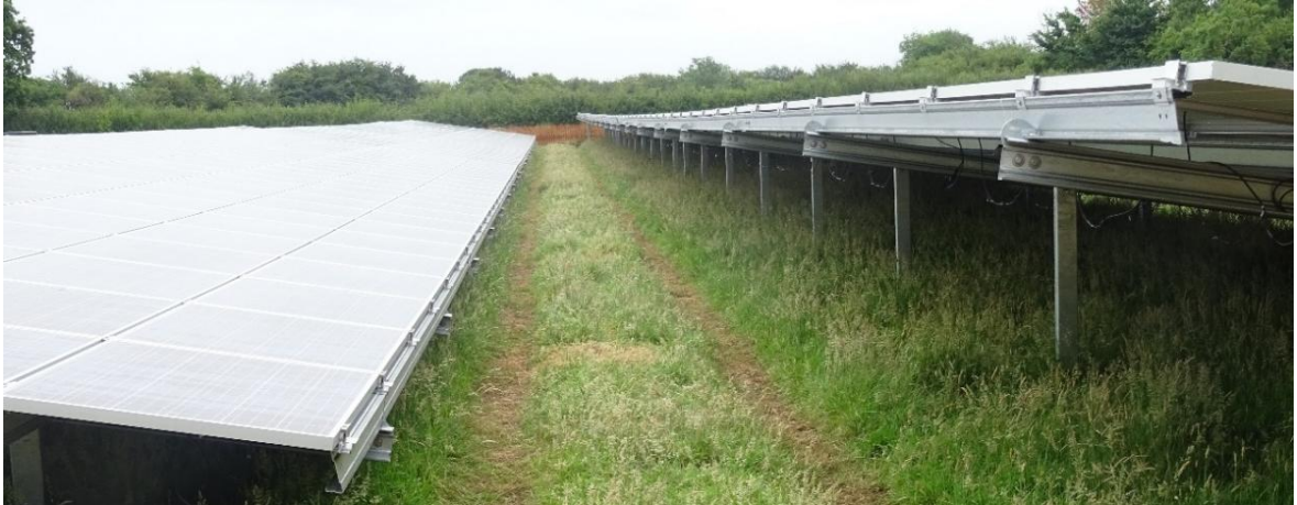
Plate 11-29 Part Installed Panels (Bentham Farm, Purton)
