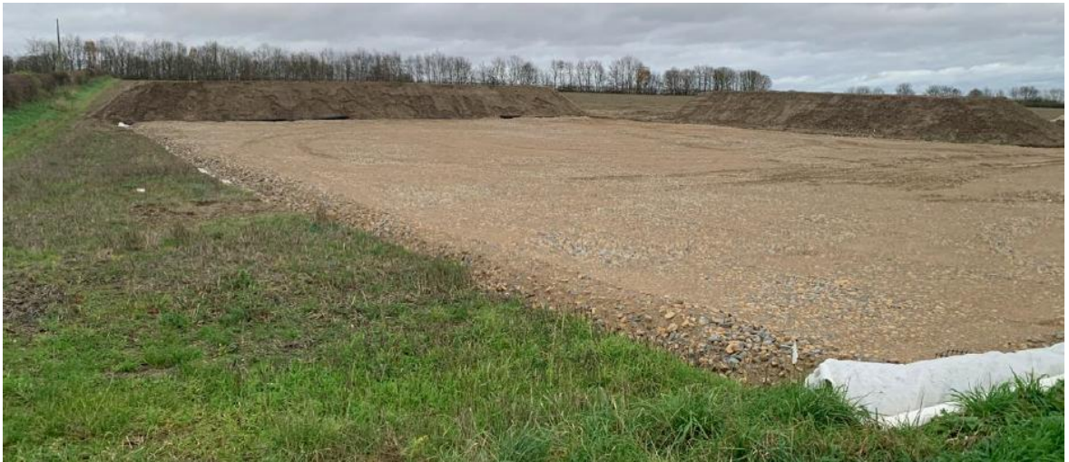
Plate 11-25 Example Construction Compound (being built)
